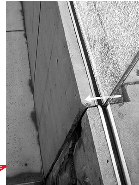
Figure 11.16. A glass guard separating Milstein Hall's loading area from an accessible ramp shattered in 2015.
