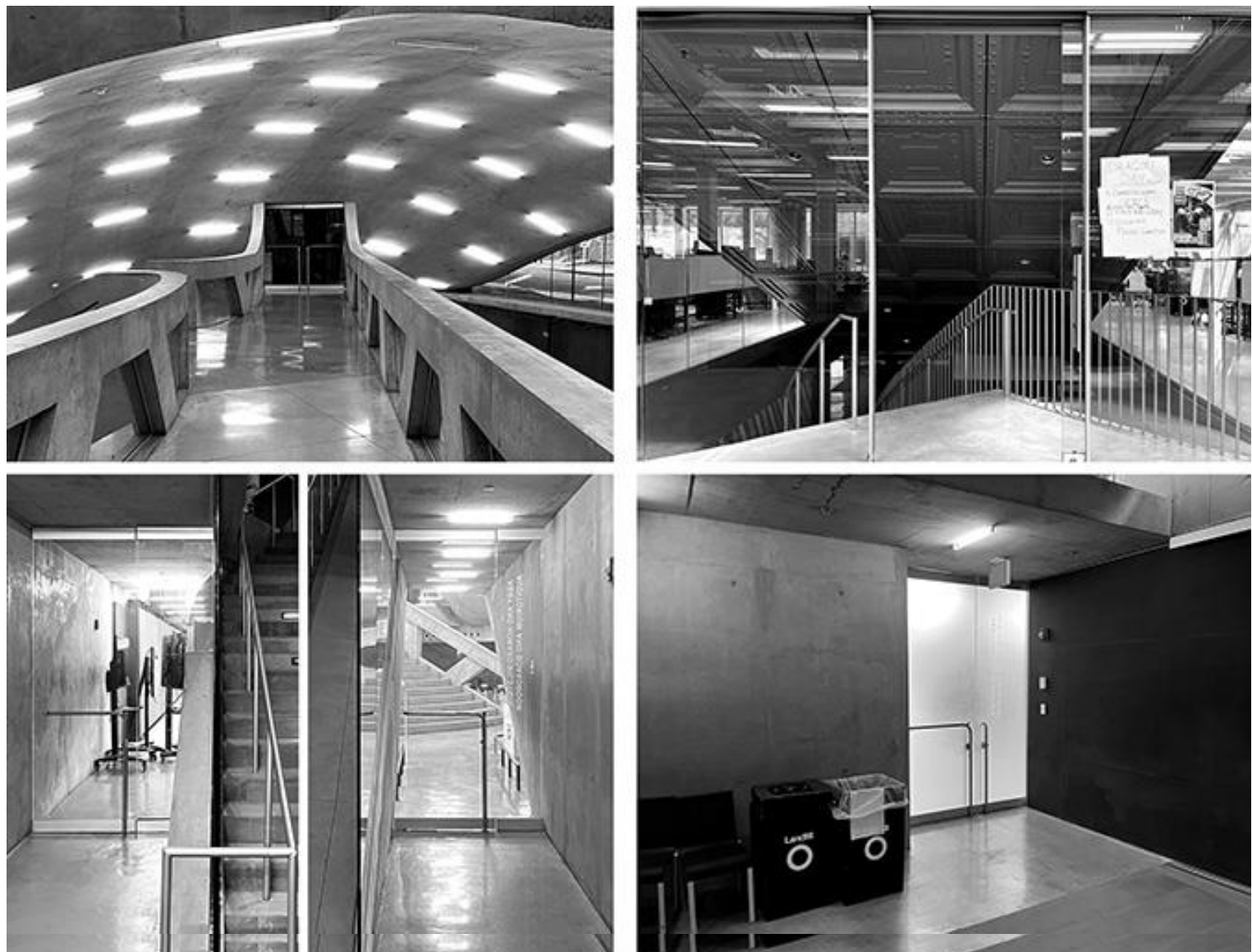
Figure 4.14. Glass doors provide no acoustic isolation for the auditorium. From top-left, clockwise: glass door from entry-level bridge; glass door from second-floor studios; glass doors into adjacent crit room; and glass door to corridor.
