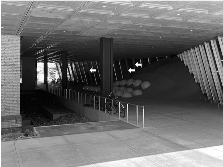
Figure 4.5. Some of the custom-designed LED lighting fixtures in the arcade that have been integrated into sloping curtain wall mullions turn themselves off for mysterious reasons, even after visits by puzzled electricians.
