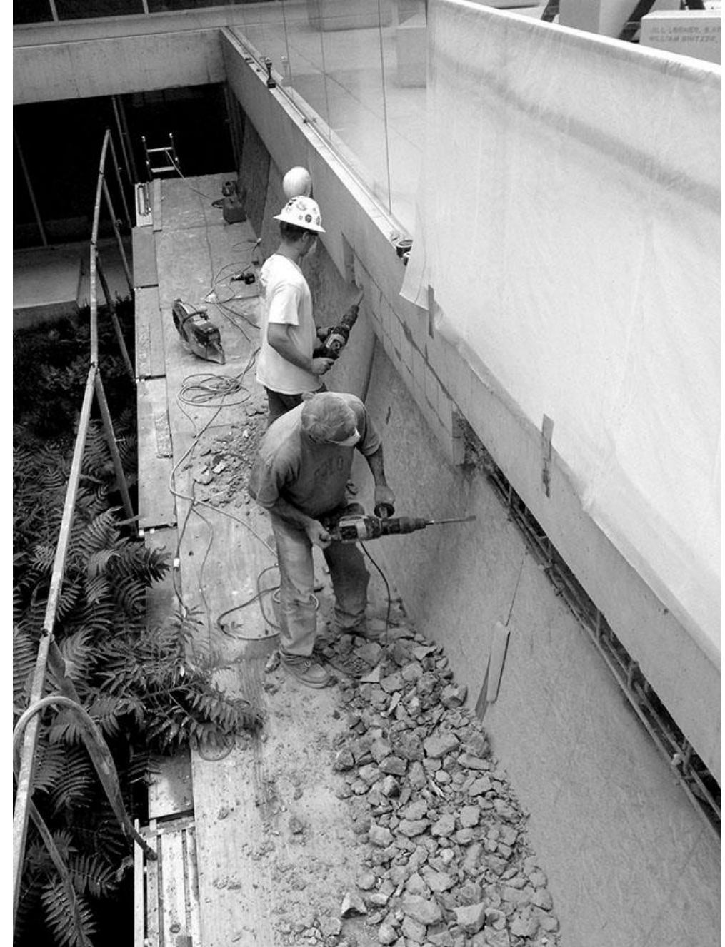
Figure 10.15. Workers remove most of the concrete fascia of Milstein Hall's Bibliowicz Gallery.
