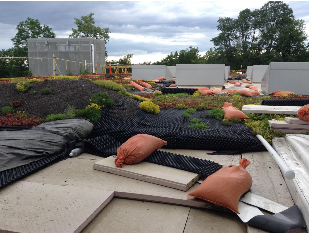
Figure 10.22. Leaks continued in 2015 (top right), triggering a major roof repair that lasted for at least two years.
