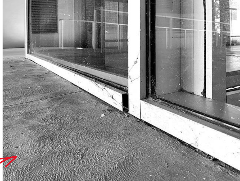
Figure 11.6. Curtain wall sill cover plates have partially or completely detached at the north side of Milstein Hall's lobby
