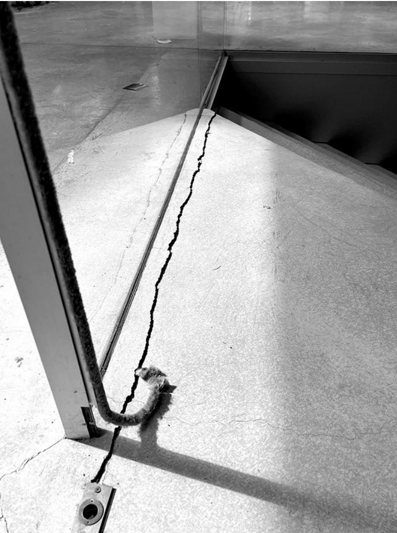
Figure 11.6. Curtain wall sill cover plates have partially or completely detached at the north side of Milstein Hall's lobby
