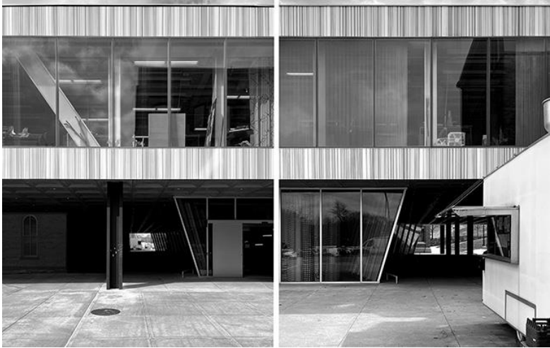
Figure 4.4. Milstein's arcade, viewed from the Milstein plaza (right) and from outside Rand Hall (left), remains dark and uninviting, even with soffit lights and integral curtain wall mullion fixtures turned on.
