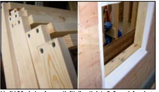
I build 26 window frames (left) directly into 2x6 rough framing in order to use vinyl replacement windows.
