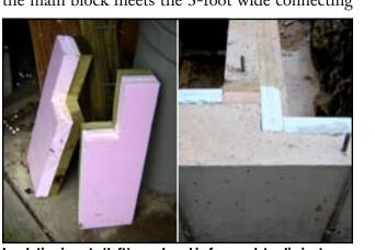
Insulation inserts (left) are placed in formwork to eliminate thermal bridge at intersecting foundation walls.
