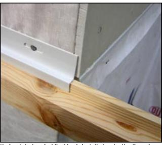
Horizontal z-bar vinyl flashing is installed under Hardipanel cement-board siding, allowing unusual "top-down" installation.
