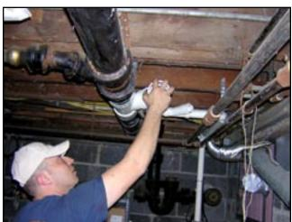
Eric Jr. connects new PVC waste line to existing cast-iron pipe.
