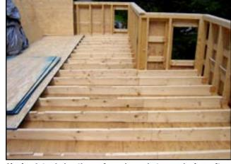
Air circulates below the roof membrane between sloping rafter spaces built above insulated joists.
