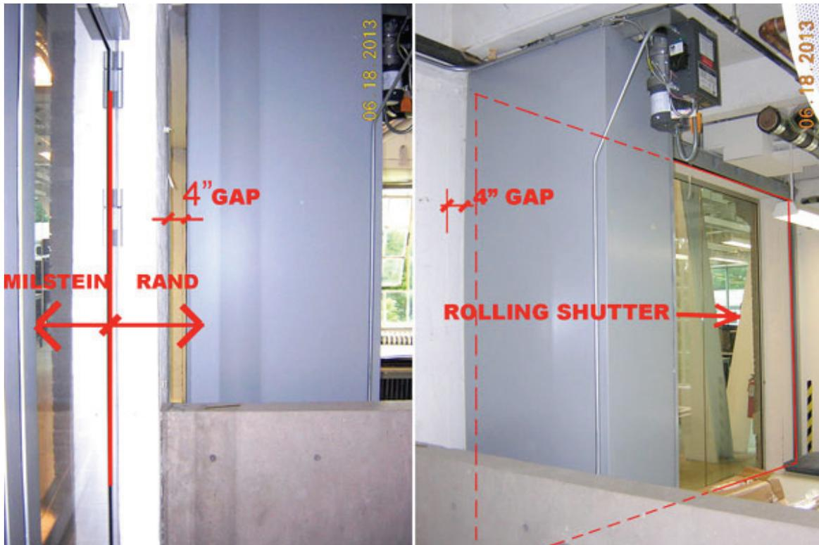
The image, taken today, shows the horizontal fire shutter in its "open" position, with the 4'-wide gap.
