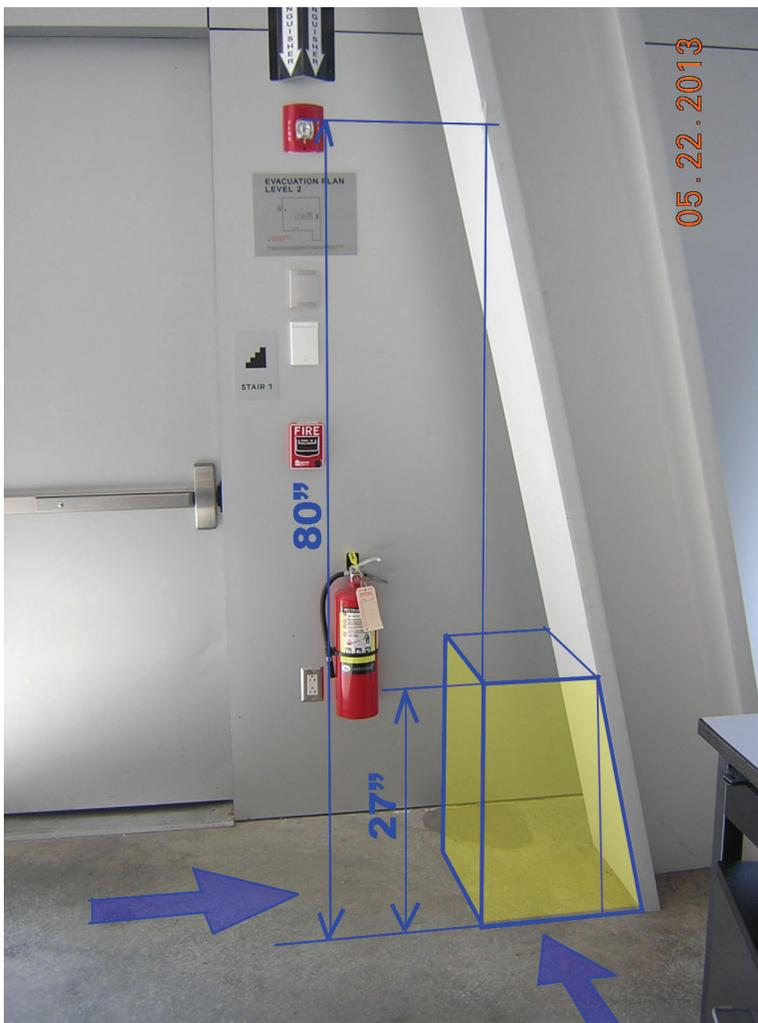
**Figure 7.** Typical angled column reducing headroom below 80 inches (labeled #1 in Figure 6). The yellow tone indicates the general area within which a barrier is needed. Photo and annotations by Jonathan Ochshorn.
